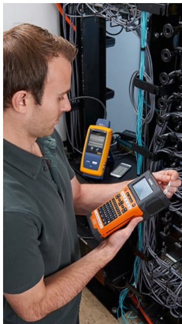
Figure 2. Labeling tools can access the identifiers in the SaaS database to save data re-entry and eliminate labeling errors.
